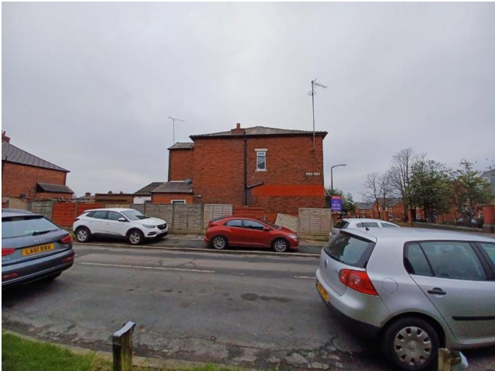
Photo 3: Side elevation of existing property, taken from Bedford Avenue.
