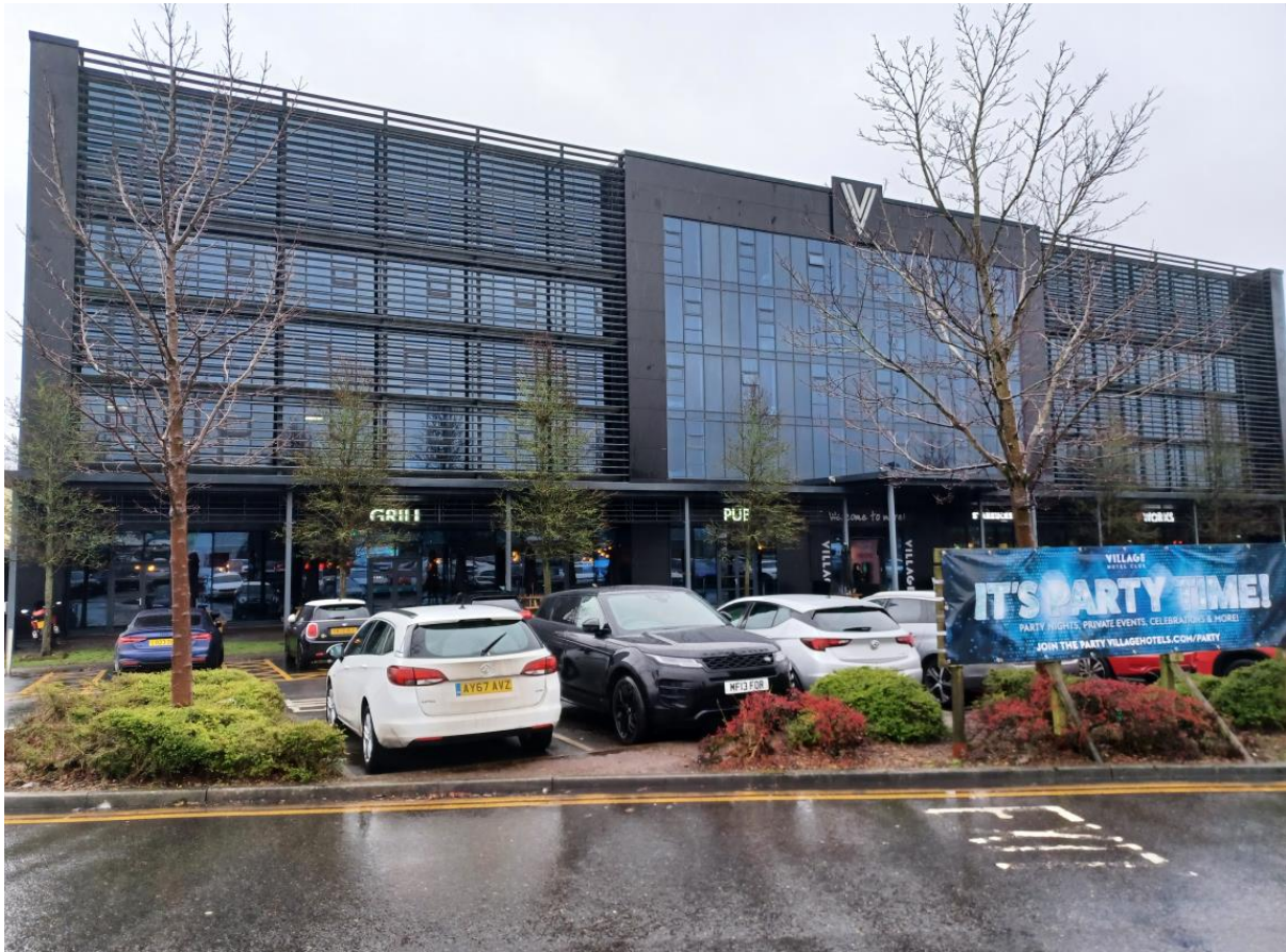
Photo 2: View of front of existing building
